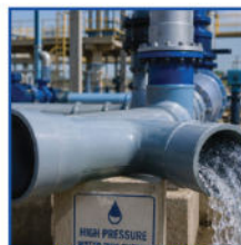
INDUSTRIAL PVC PIPING PROJECTS
